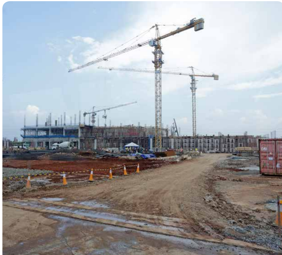
Konstruksi AEON Mall, BSD City/ The Construction Of AEON Mall BSD City
